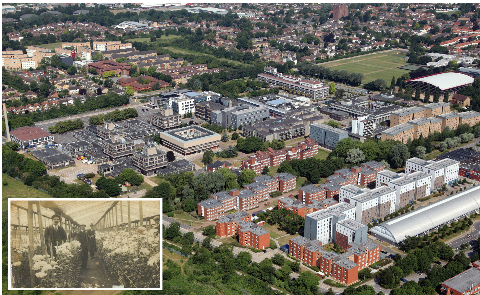
■ Main picture: an aerial photo of the Brunel University of London campus in the 21st century. Inset: inside one of the many glasshouses that stood on the site in the first half of the 20th century
